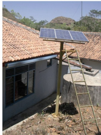
A small solar array of 180 watts can power this solar direct-drive vaccine refrigerator.
