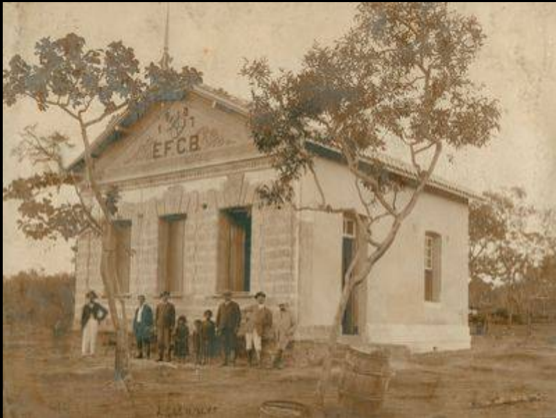
Chagas (the second on the left) at a building of the Central do Brazil Railway in Lassance COC Archives.
